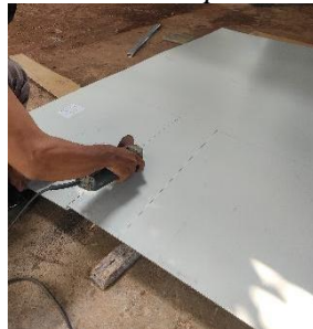
Gambar 10. Proses Pemotongan Aluminium Composite Panel (ACP)
